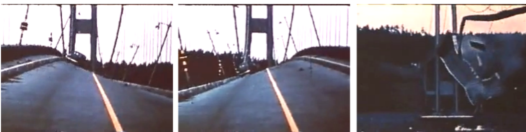
Figure 1.2: Collapse of the Tacoma Narrows Bridge (1940).
