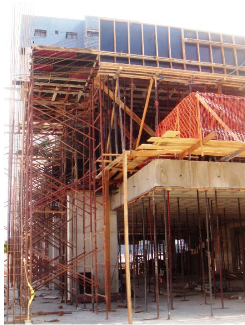
Figure 1 – Scaffold system in Fortaleza-Brazil.
