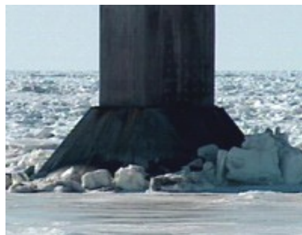
Figure 3. Ice impacting with pier, Confederation bridge
