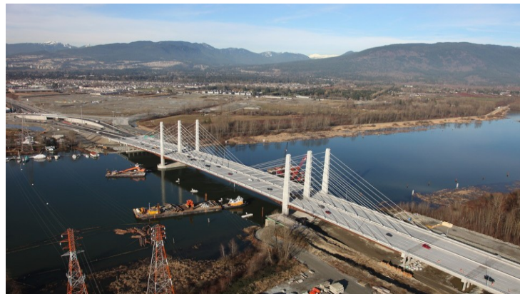
Figure 5. Pitt River bridge, British Columbia, 2010
