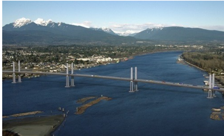
Figure 4. Golden Ears bridge, British Columbia, 2009
