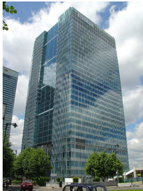
Figure 2: Barclays Bank Head Office, London, UK (Lytag, 2013).
