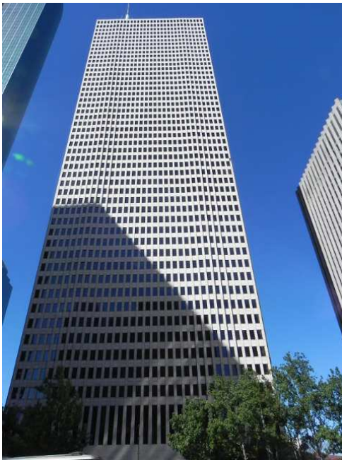
Figure 1: One Shell Plaza Tower, Houston, USA. (Khan, 2004)
